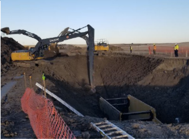
Digging ditch - km 195+580 – Oct 27, 2018
