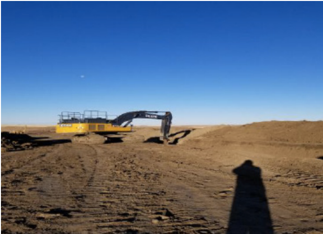
Excavator digging ditch - km 193+050 – Oct 27, 2018
