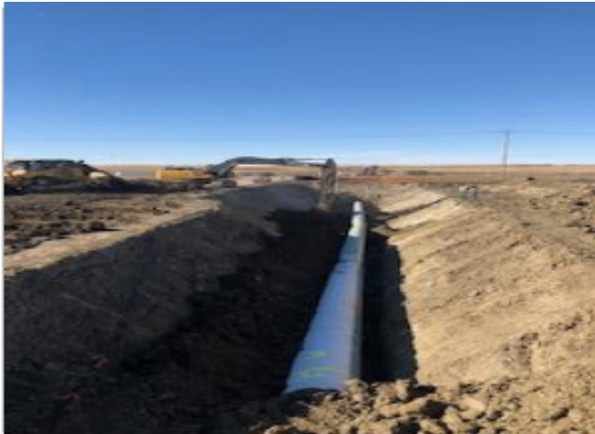
Tie-in backfill – km 170+880 – Oct 26, 2018
