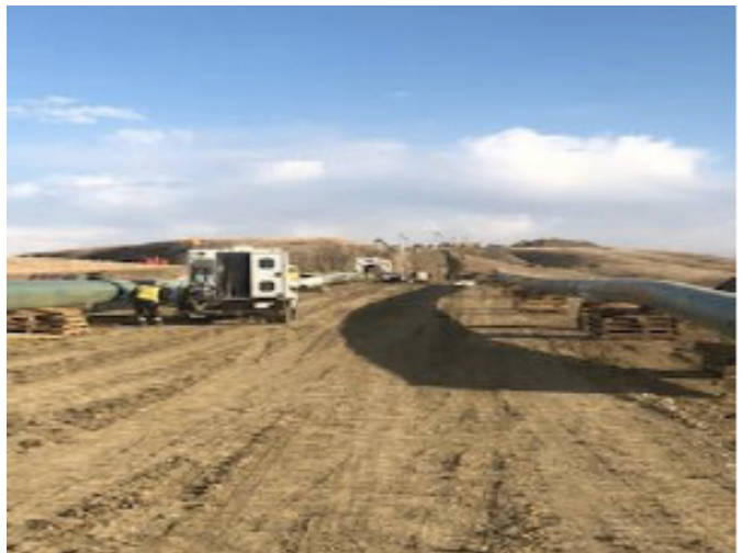
Last weld – km 222+600 – Oct 25, 2018
