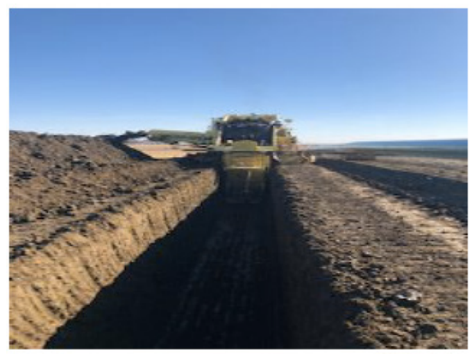
Wheel ditcher digging mainline – km 194+600 – Oct 23, 2018
