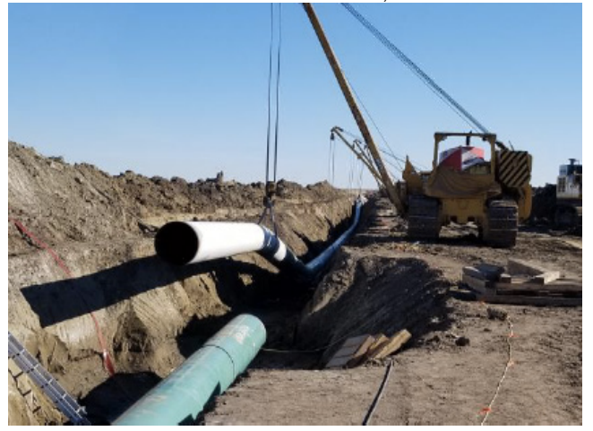
Welding tie-in section – km 155+800 – Oct 22, 2018
