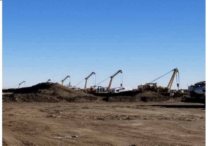
Excavator moving spill pile – km 255+180 – Oct 26, 2018
