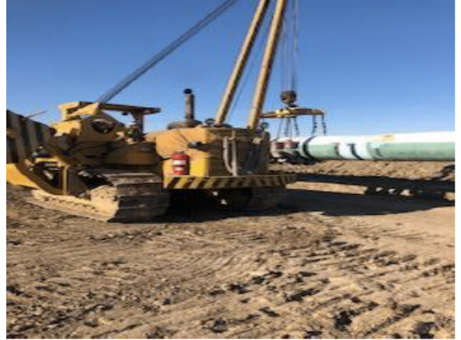
Lower-in crew – km 189+300 – Oct 22, 2018
