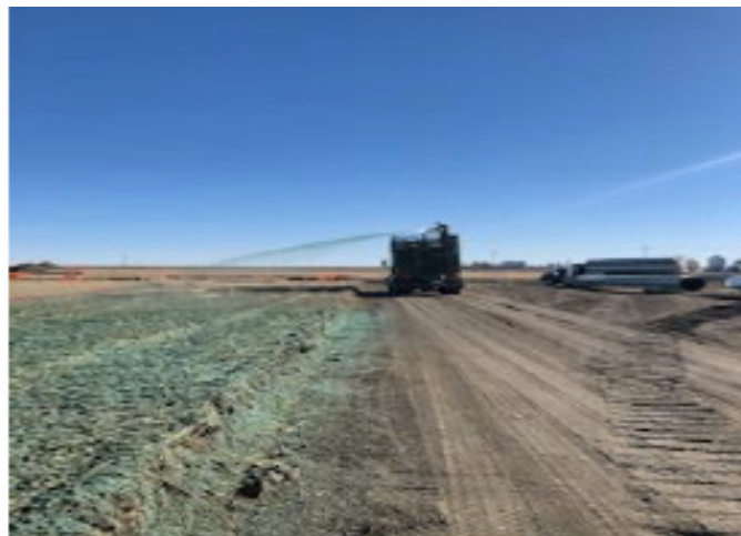
Hydro mulch being sprayed – km 223+400 – Oct 22, 2018
