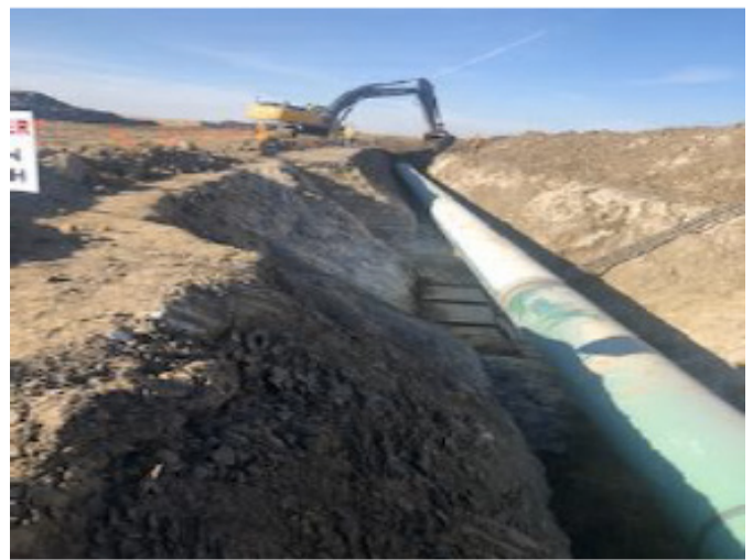
Shading tie-in ditch – km 157+430 – Oct 24, 2018
