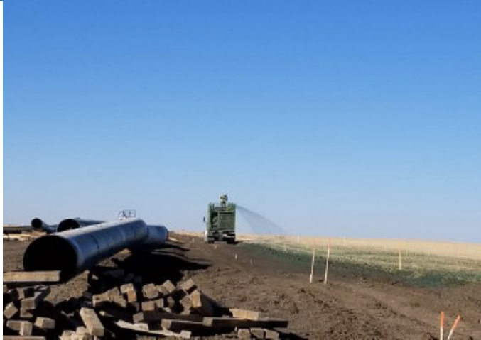
Hydro mulch - km 238+170 – Oct 26, 2018
