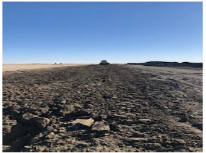
D6T following backfill excavators – km 201+112 – Oct 27, 2018
