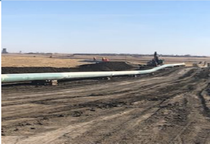
Laying geotec for ditch – km 192+700 – Oct 23, 2018
