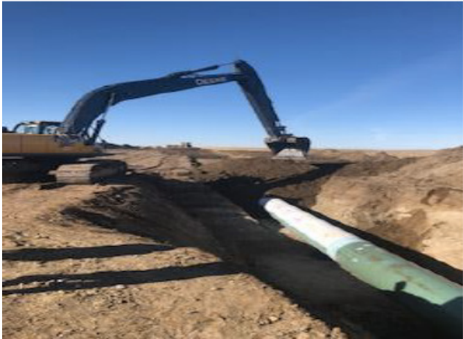
Excavator shading final tie-in backfill – km 155+700 – Oct 22, 2018
