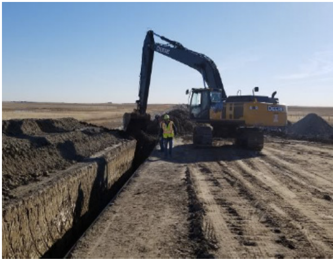
Shading pipe – km 156+250 – Oct 23, 2018
