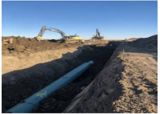
Backfill tie-in (south) – SF 111– Oct 26, 2018
