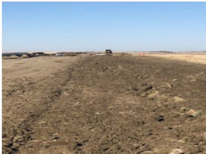
Dozer shaping mainline ditch– Km188+950 – Oct 23, 2018
