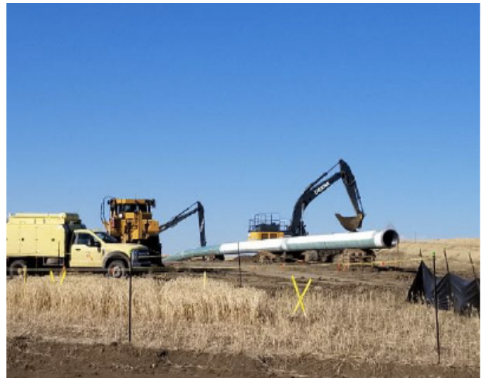
Digging ditch and crumbling ditch– km 192+800 – Oct 23, 2018
