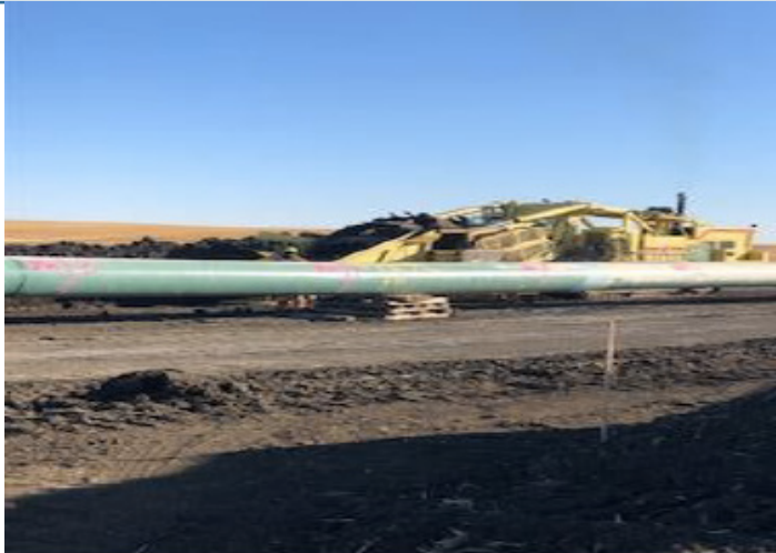
Ditching wheel working through wetland – km 197+850 – Oct 24, 2018
