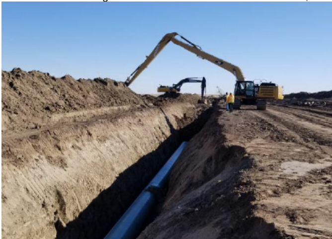
Backfill pipe – km 155+600 – Oct 22, 2018
