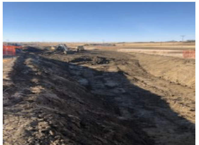
Cutting on ROW for bore crew – km 196+370 – Oct 22, 2018
