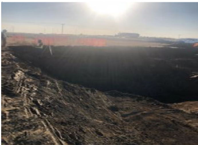
Bore bay being dug – km 259+100 – Oct 25, 2018
