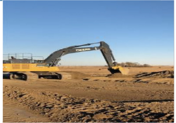
Excavator cleaning spill pile– km 159+250 – Oct 23, 2018
